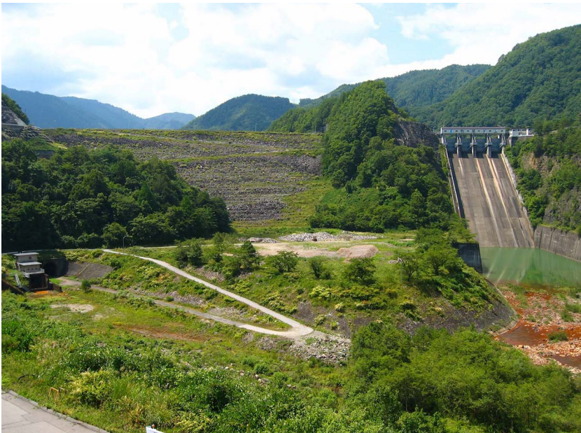
Figure 1 ■ Makio Dam (creative commons license: https://commons.wikimedia.org/wiki/File:Makio_Dam.jpg )
